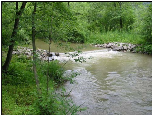
Stream habitat improvement project on Cherry Run
