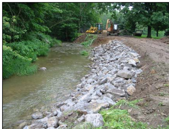
Streambank stabilization project at Falcon Park, construction phase, June 2003
